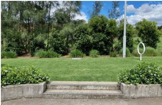
2 EXISTING STAIRS LEADING INTO SITE TO BE REPLACED WITH NEW RAMP AND LOW WING WALLS RETAINING TURF
